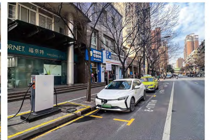
The first on-street parking EV charging station in Shanghai, China 🇨🇳
