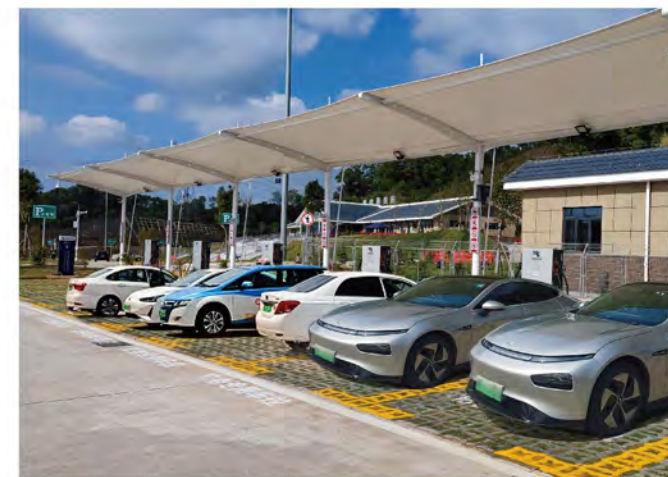
Highway service area EV charging station in Shenzhen, China 🇨🇳
