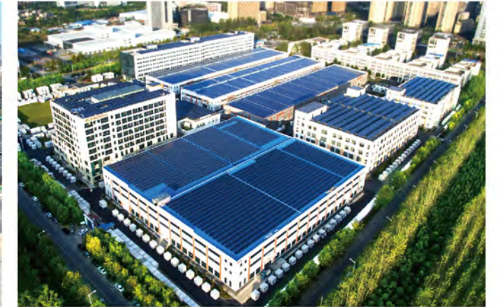
PV+ESS+Charger station in Sungrow HQ in Hefei, China 🇨🇳
